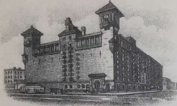
52 ND STREET BUILDING
