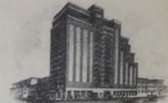
80 TH STREET BUILDING
