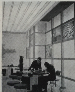
Ceiling in cafeteria of Northport school has gaily colored fixtures on dropped panels. Fluorescent tubes atop edges of panels light cellular decking above which is bright orange
