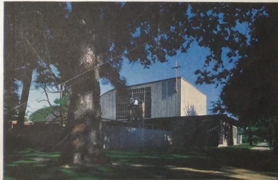
Architect Belluschi used native timber to create a house of worship which also meets the social needs for Cottage Grove, Oregon's, First Presbyterian Church.
