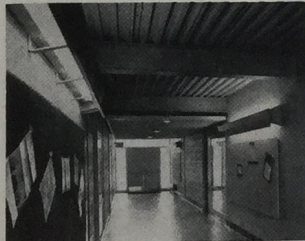
Same school as above uses wood baffles in front of fluorescents to light display board and corridor. Downlights are in dropped ceiling for entrance
