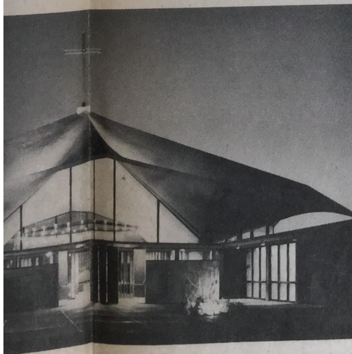
Built on a hilltop, the Mercer Island, Washington, Presbyterian Church is a beacon at night. The walls are of plate glass. The concrete roof is meant to suggest cupped hands up-lifted.
