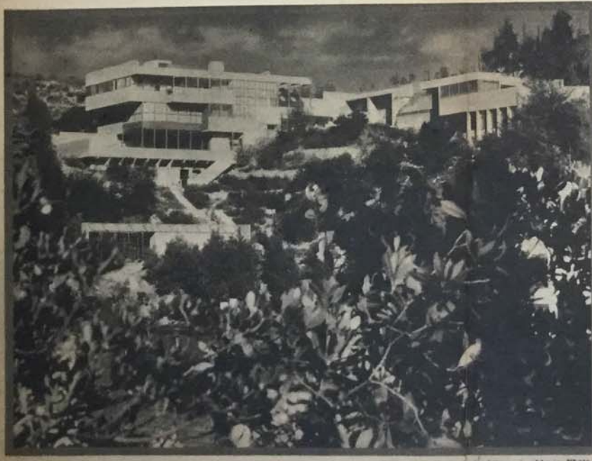
New Architecture for Dwelling—A Steel Construction House in Los Angeles.
