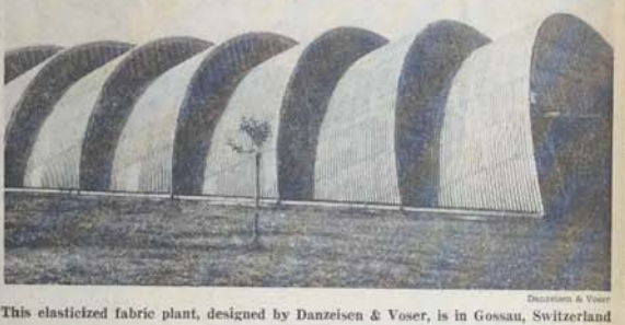
This elastized fabric plant, designed by Danzeisen & Voser, is in Gossau, Switzerland.
