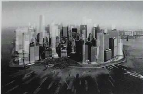
Architecture Research Office and dlandstudio's New Urban Ground transforms Lower Manhattan with an infrastructural ecology. [Image credit: Architecture Research Office and dlandstudio]
