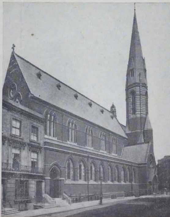
St. Mary Magdalene's, Paddington (architect, G. E. Street)
