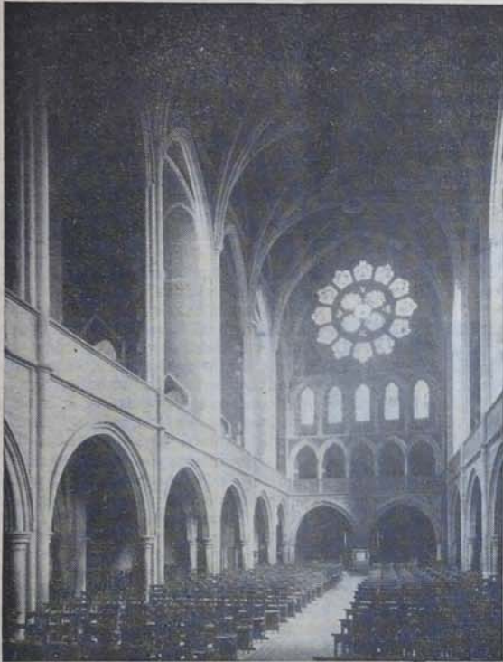
St. Augustine's, Kilburn (architect, John Loughborough Pearson), showing part of the triforium passage at 'first-floor' level
