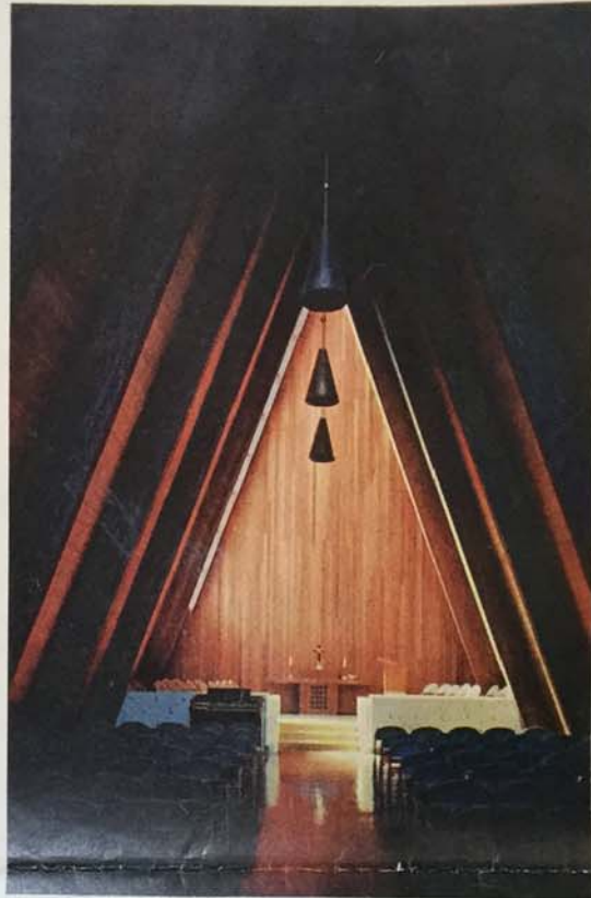
LAMINATED BEAMS of fir support steep roof, finished in hemlock, of the Congregational Church in Cedar Hills, Ore. Designed by Warren Weber, church cost $45,000, seats 155.
