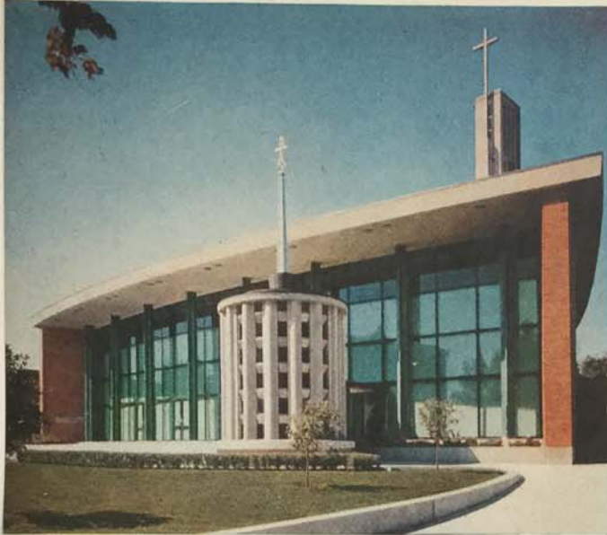
PARABOLIC PLAN was used in Catholic Church of the Resurrection in St. Louis, whose walls follow parabola's curve. Glass front, with round baptistry, stretches between ends of wall. Inside (below), a halo of light floods altar and mural based on Apostles' Creed. Architects were Murphy and Mackey.
