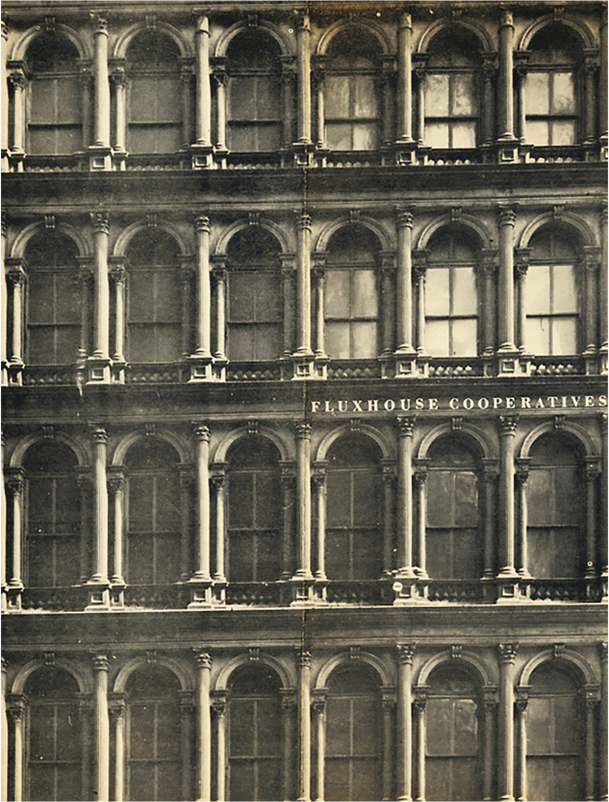
Fluxus Cooperative Building Project, 1966. More ►
