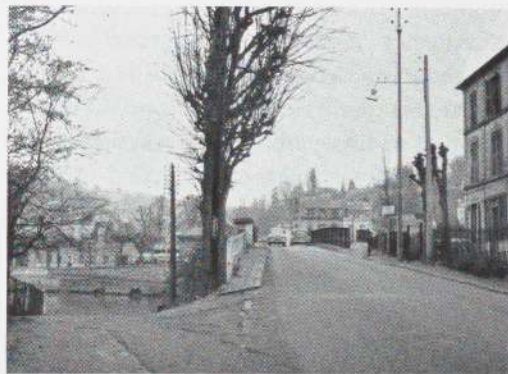
View across the bridge toward Bougival. (Photograph, 1958)
