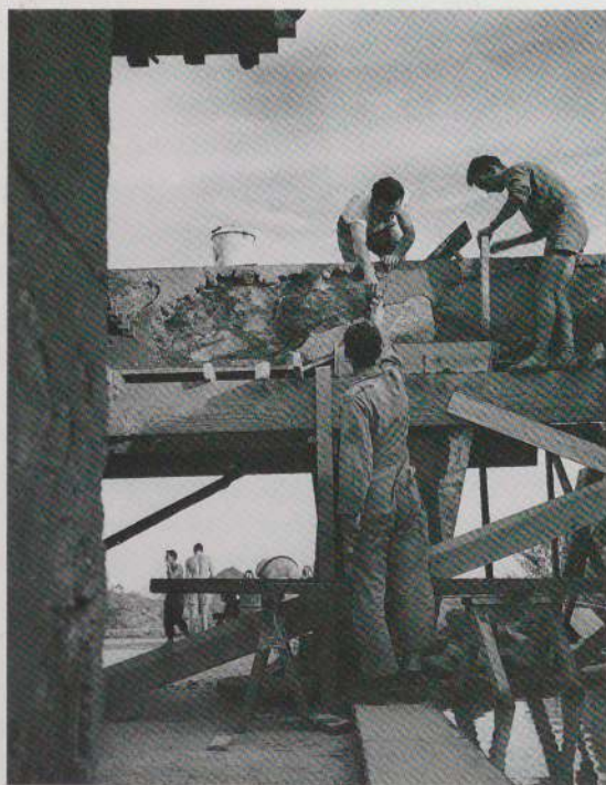
Figure 10: Frank Lloyd Wright. Taliesin West, Scottsdale. 1937–38. Under construction
